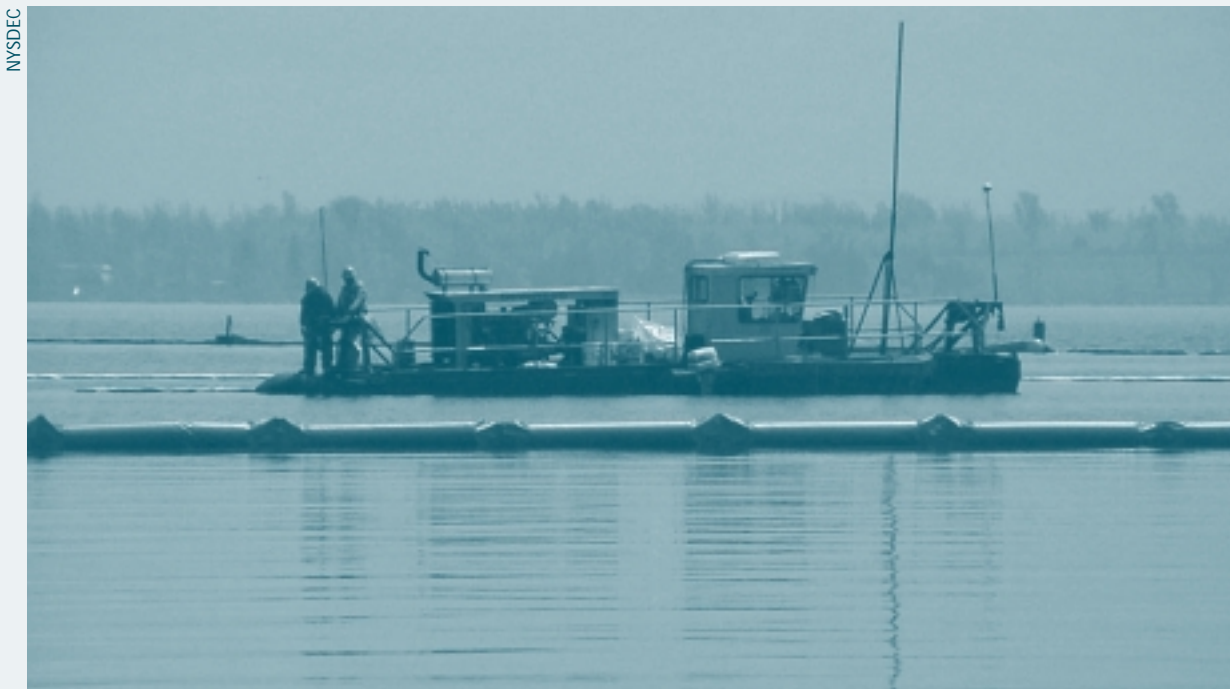
The Cumberland Bay cleanup, led by the NYSDEC, removed 140,000 tons of PCB-contaminated sludge from the Bay.
