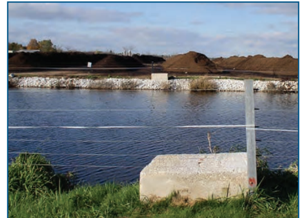
NRCS built this waste storage pond at Foster Brothers Farm in Middlebury, Vermont, to collect phosphorus runoff from compost.
