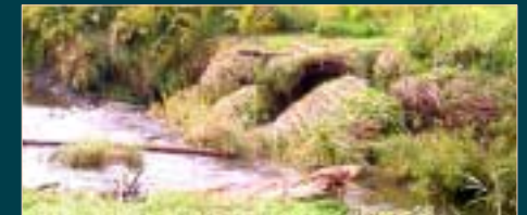
Unforested riparian areas result in instability and erosion along many of Vermont's rivers and streams. This slumping streambank along the upper Winooski River could be helped with a riparian buffer of trees and shrubs.
