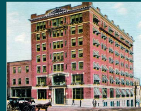
At seven stories, the Hotel Vermont, located at the Park's southwest corner, is still one of Vermont's tallest buildings. Built in 1910 in the Colonial Revival style, the building featured a glazed roof garden and wrought iron seventh story balconies to take advantage of views of the lake and park.
