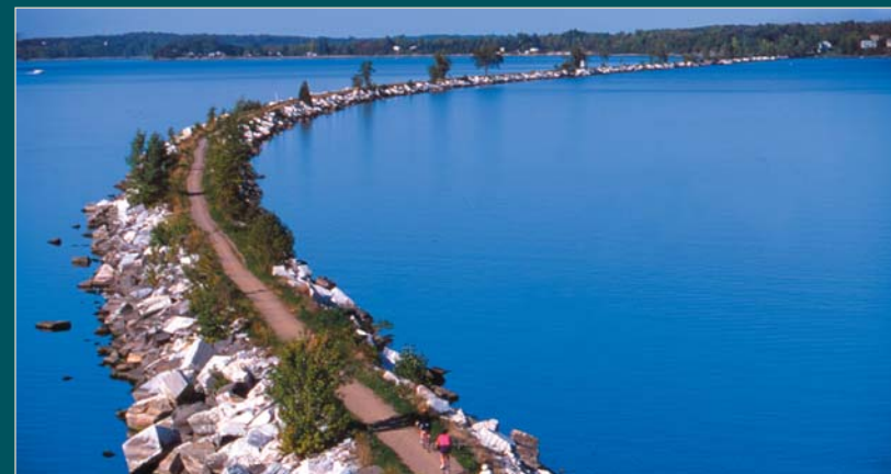
Over 598,000 cubic yards of fill and marble "armor stone" was needed for this engineering achievement. To limit the amount of fill needed, the causeway was built on the shallowest depths, which explains its curved alignment.
