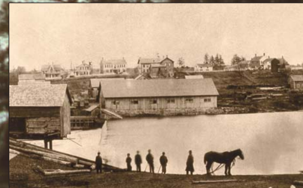
From the late 1700s to the early 1900s milling lumber was an important industry in Winooski. Logs cut upstream were floated down river to Winooski where they collected in the pond behind the dam at the upper falls. There workmen hauled them out and milled them on saws powered by water. In the early days the finished boards were stacked on large rafts and floated down river to Lake Champlain and then to Québec. Later most of the wood was used locally, in the construction of furniture, window frames and doors. (This image and main image of Winooski courtesy of the Winooski Historical Society.)
