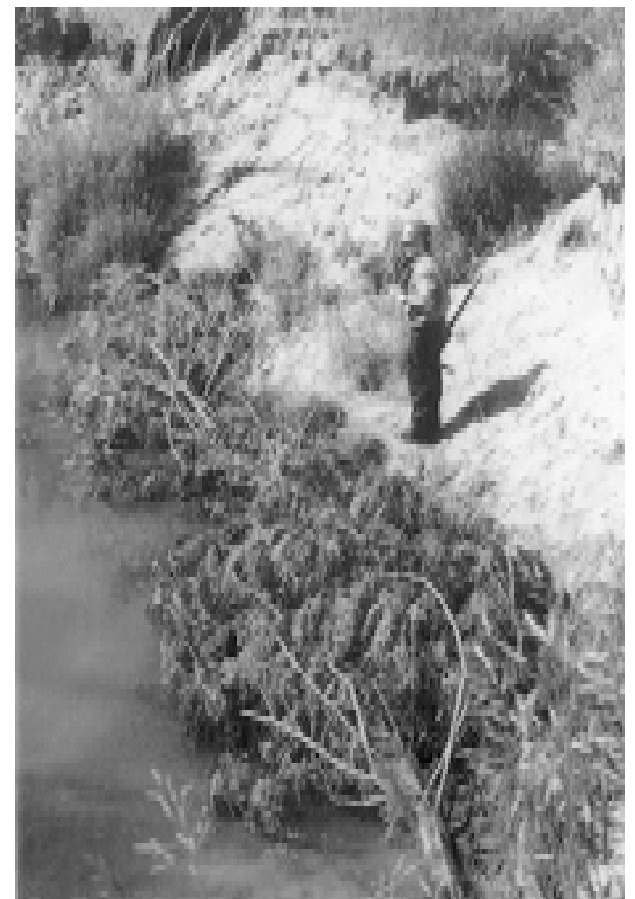
A Vermont Youth Corps member working on a streambank stabilization project.
