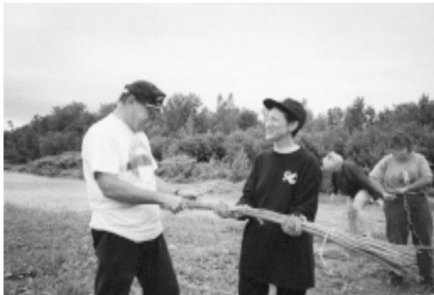
Preparing willow waddles for a streambank planting.
