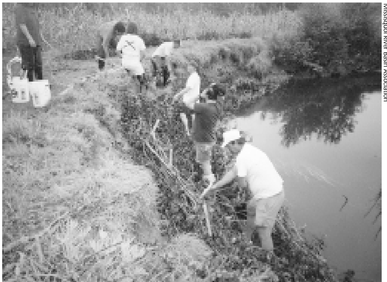
Stabilizing a streambank in the Missisquoi Basin.
