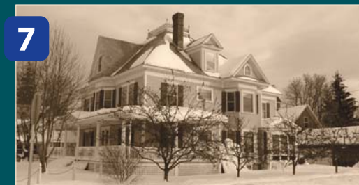
7 Marvin House (ca. 1900) - This home is a fine example of Colonial Revival architecture. Its materials came from a variety of Vermont sources: wood from Underhill and Jericho, red rock foundation stone from Burlington and roof slate from Rutland County.
