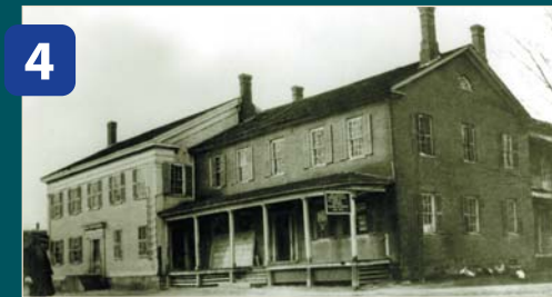
4 Lincoln Hall (1819) - Its right side was built first in Federal style while the left side is Greek Revival from the mid-1800s. It was a tavern until 1911. The Village bought it and used it as a library, hardware store and a residence. Today it serves as the municipal offices.
