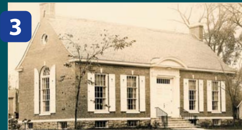
3 Brownell Library (1926) - A gift from Samuel Brownell, a prominent local businessman who developed hydroelectric power, it was described as "in every sense a Vermont building" with its foundation of redstone, a roof of unfading black slate and white marble sills and columns.
