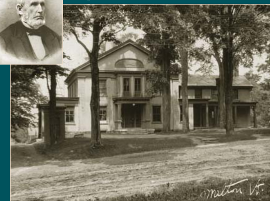
Built in 1835, the Joseph Clark residence on lower Main Street was deeded to the town in 1919. Known as the Clark Memorial Building, it housed the town offices until 1994.
