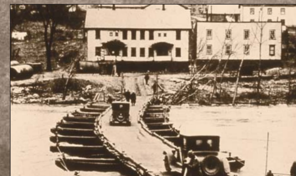
With the old bridge gone, the U.S. Army Corps of Engineers erected a temporary pontoon bridge to get people across the river. Can you imagine walking across it as it as it bobbed up and down on the water—almost like being on a roller coaster. (This photo and main image of flood courtesy of the Winooski Historical Society.)
