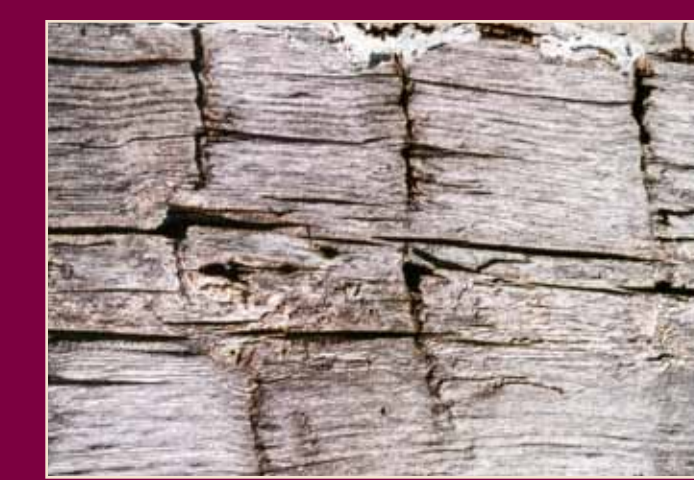
Recent views of the exterior of the 1797 log cabin show that the broad ax marks are still visible after more than 200 years. The interior reveals the rickety staircase to the loft where the family would have slept. Photos courtesy David Patrick.
