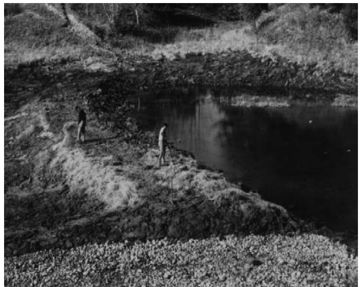
Wetland Restoration, Senn property, Essex Junction, VT.
