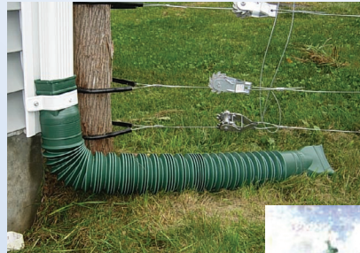
Top: Example of a downspout extension
