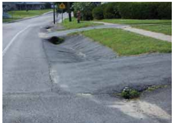
Keeseville, NY. Fast, paved ditches can be replaced with slow, vegetated swales, using drainage easements on private land if necessary.
