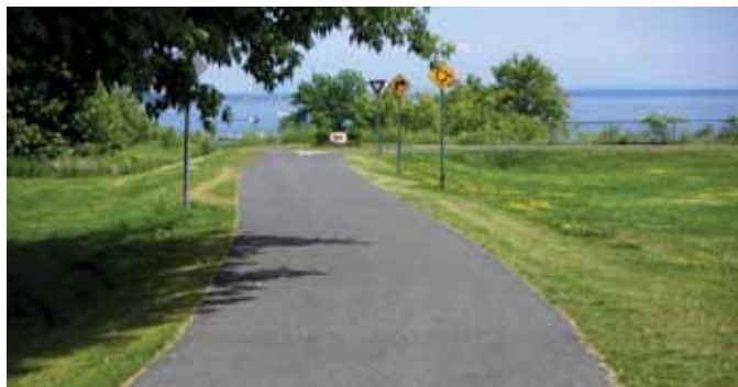
Plattsburgh, NY. Stormwater from walkways and bicycle paths often can be managed simply with a well-designed buffer.
