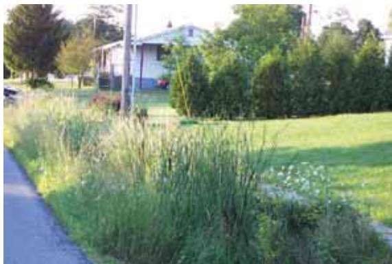
Vergennes, VT. Distributed stormwater management practices can reduce the need for more costly centralized practices. This vegetated swale functions to slow, store, and treat stormwater.
