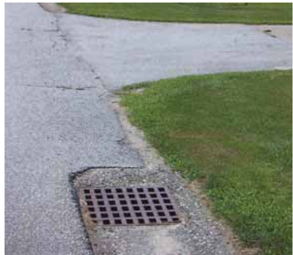
Wallingford, VT. The relative presence or absence of storm drains is one indication of how well green space is being used to manage stormwater.
