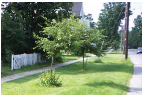
Bristol, VT. Vegetated buffers allow stormwater to spread out and infiltrate into the ground.
