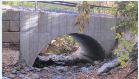
The completed project with natural substrates.
