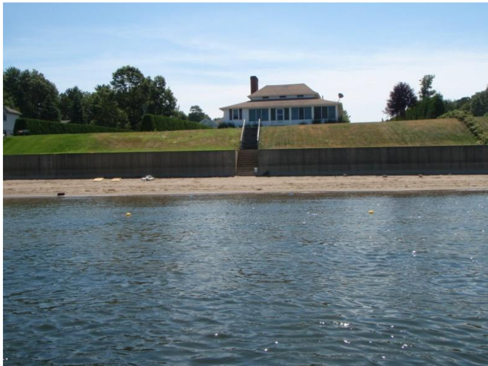
Figure 3.5: Bank armoring and intensive shoreline development in Malletts Bay.
