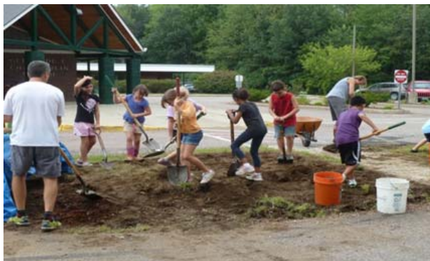
Students work on a rain garden construction project.
