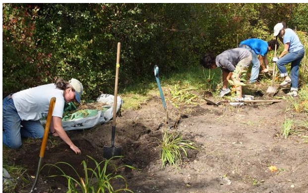
Newly armed with stormwater management knowledge, homeowners construct a rain garden.
