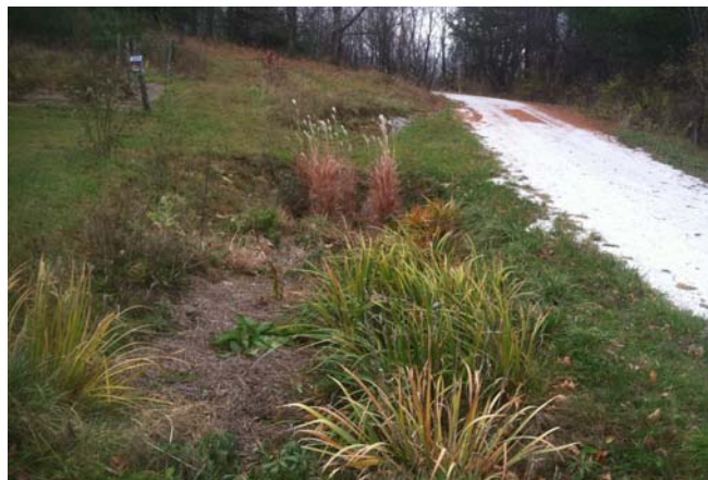
Rain garden installed in Shelburne, VT as part of BLUE certification.
