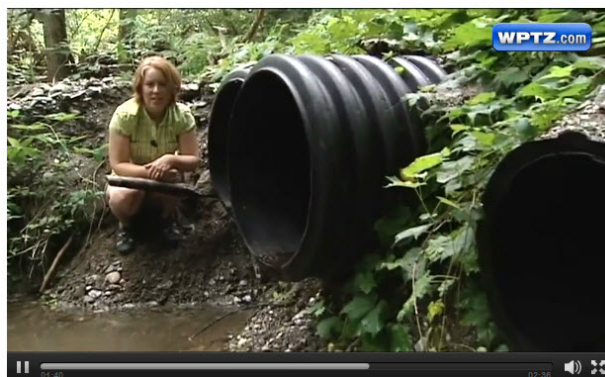
Conservation Correspondent Bridget Butler reports on impassable culverts for WPTZ.
