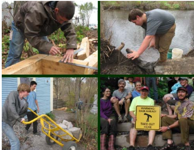
Creating river access sites.
