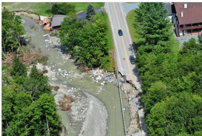
A segment of Route 100 destroyed by Irene.
