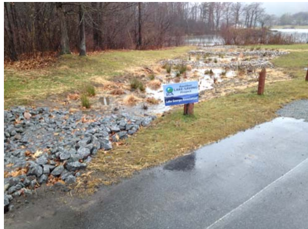
Pocket wetlands catching runoff from their first rain event post-installation.
