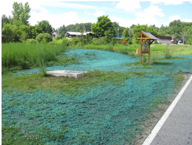
Hydroseeding at West Brook in Lake George Village.
