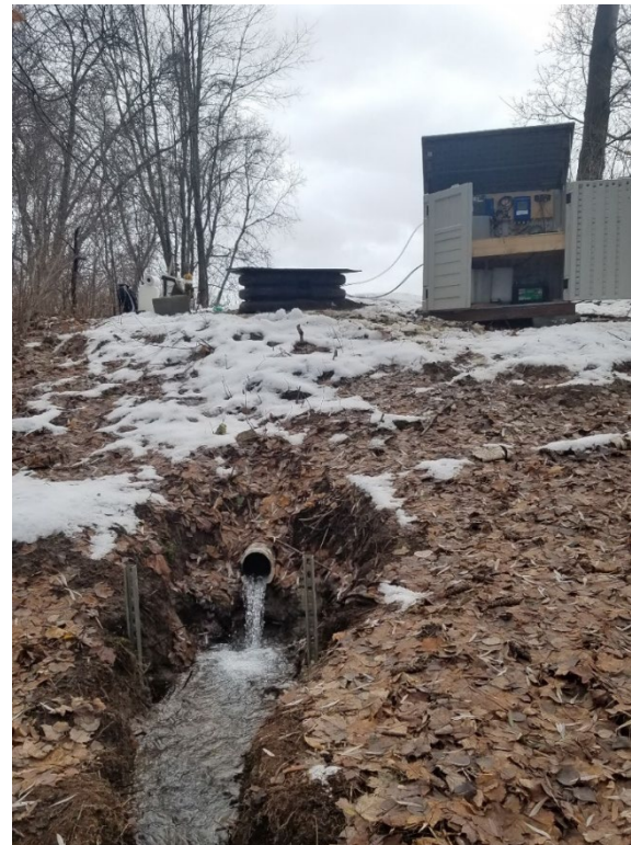
Figure 29. ACT1 tile drain outlet
