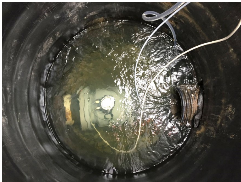
Figure 7. 8-inch Waterflux 3000 flowmeter in JBT11 manhole
