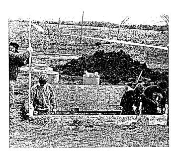
Prior to installation of the sand filter, the failed mound was removed. A foundation footing drain which had contributed to the failure was isolated from the wastewater treatment systems. A conventional mound for dispersal of the effluent was constructed to blend with the topography created by a house addition. Imported sand and stone fill was necessary to obtain the required 36" separation distance to groundwater.
