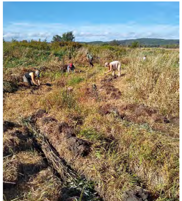
Fascine and live stake installation at a site in Cornwall in 2021. These areas had been prepped by clearing competing vegetation ahead of install, creating easier access, more efficient digging, better site conditions for establishment next season.
