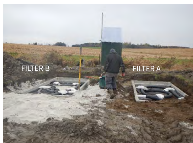
Phosphorus filters filled with media, prior to placing on lids. Filter B (left) was comprised of limestone “bedding sand” and Filter A (right) contained drinking water treatment residuals.
