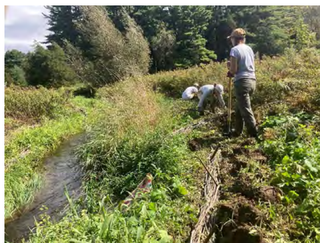
Fascine and live stake installation at a site in Poultney, VT
