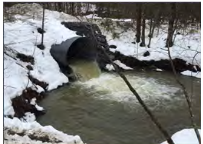
Purchase Brook culvert with roughly 2' drop to water surface at outlet and high levels of scour downstream of the culvert.
