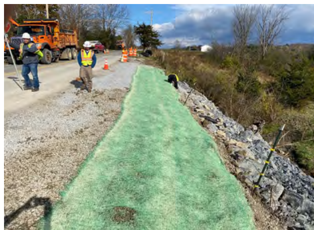
Stabilization of the road bank on the Winchell Creek side utilizing rolled erosion products, woody vegetation, hydroseeding, and hardscaping
