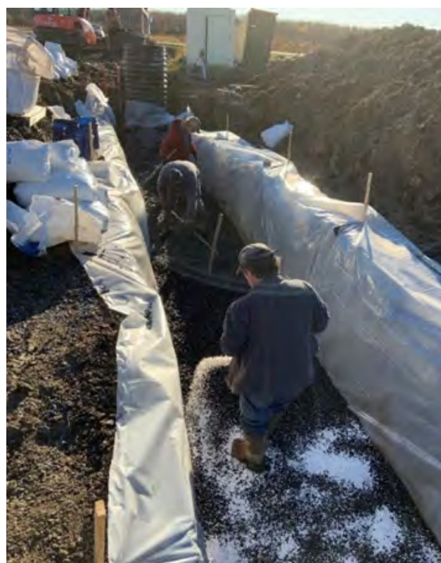
Constructing a P filter at the outlet of a tile drain in St. Albans
