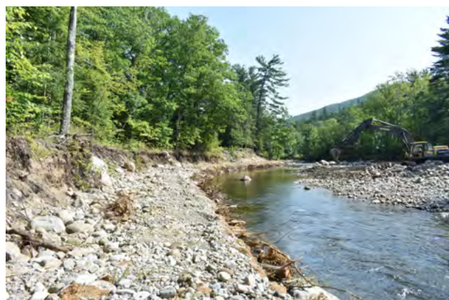
Completed toe wood bench from Figure 8. Photo looking downstream from top of bench.
