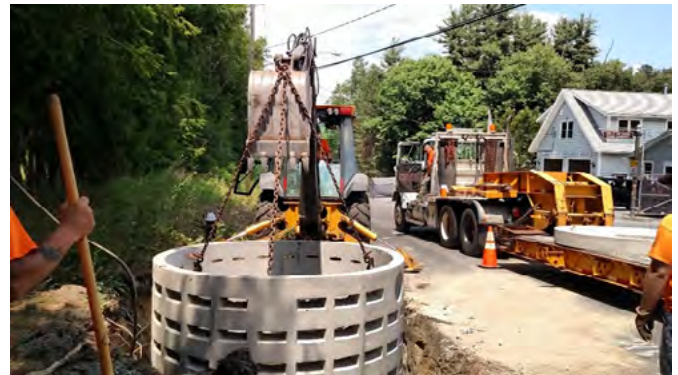
Image of a dry well getting installed on a previous Lake Champlain Basin Program funded project in the Town of Lake George. The Town of Lake George Highway Department installed the structure.
