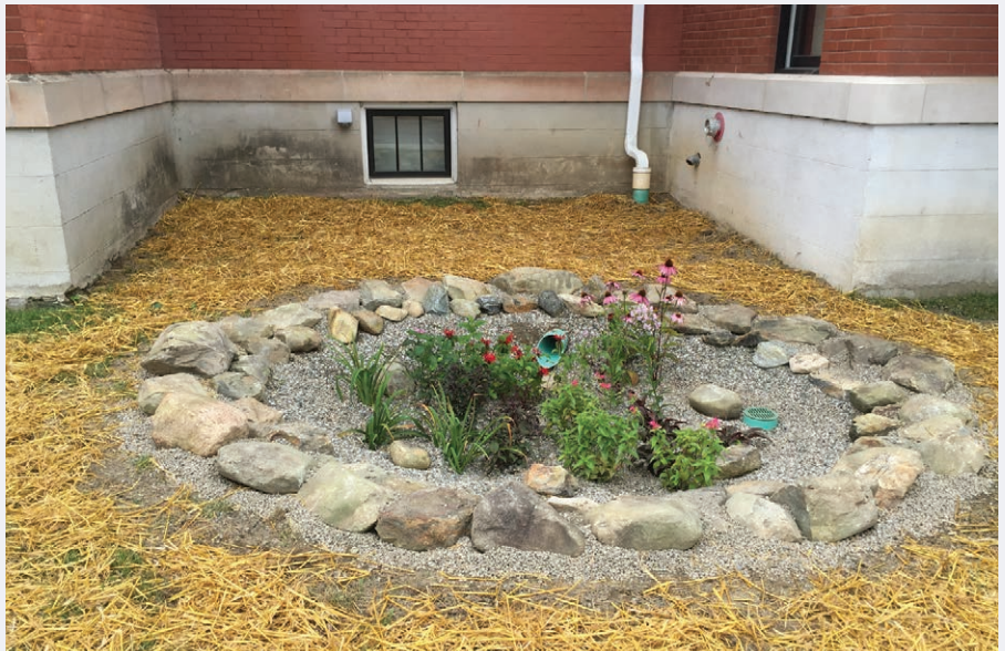
Image 5-CS-5-1. Newly-installed rooftop runoff rain garden. Stones instead of mulch were used as mulch will float and move around (and contains phosphorus, which can be exported into groundwater).
