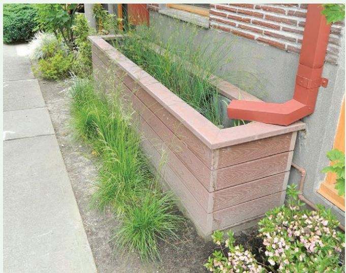
Image PE-18-2. Photo of a simple downspout connection to a stormwater planter.
