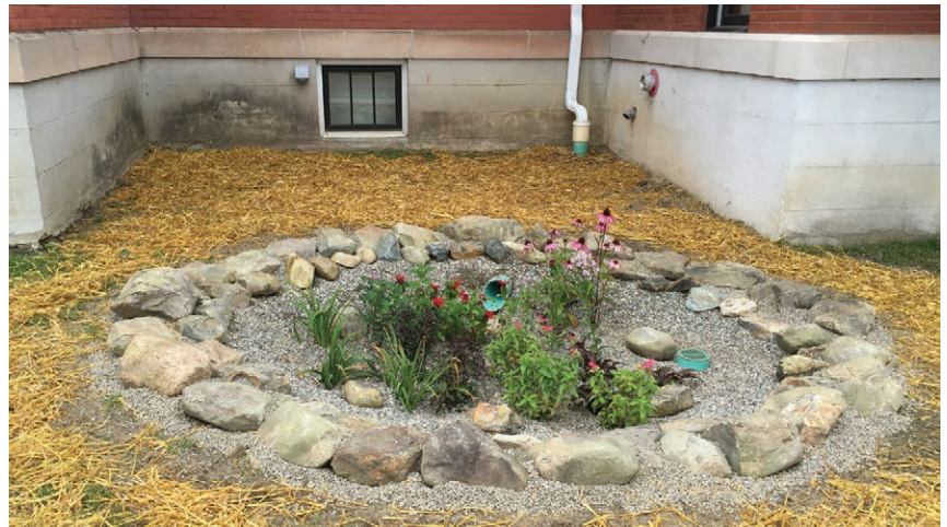
Image 5-2. A simple rooftop runoff rain garden at the Morrisville Public Library in Morrisville, VT serves to infiltrate rooftop runoff that would otherwise spill across pavement and transport pollutants to the stormwater sewer.
