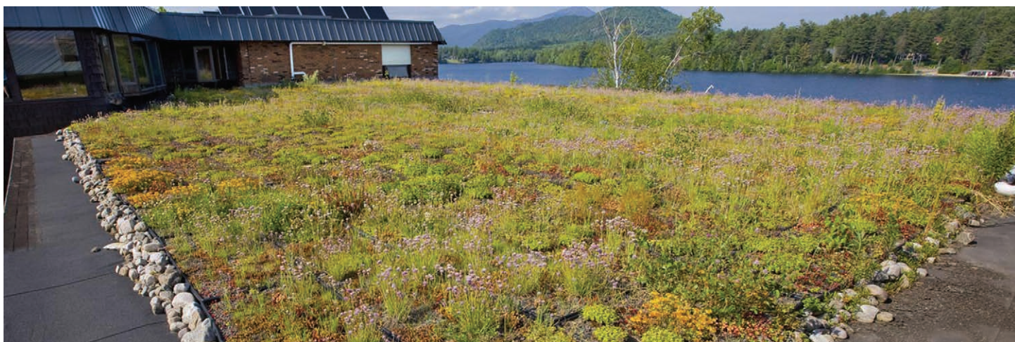
Image 5-1. Rain that falls on the Golden Arrow Lakeside Resort roof in Lake Placid, NY is collected and retained in the soil and plants on their green roof, slowing down peak discharge to stormwater sewers and natural water bodies.
