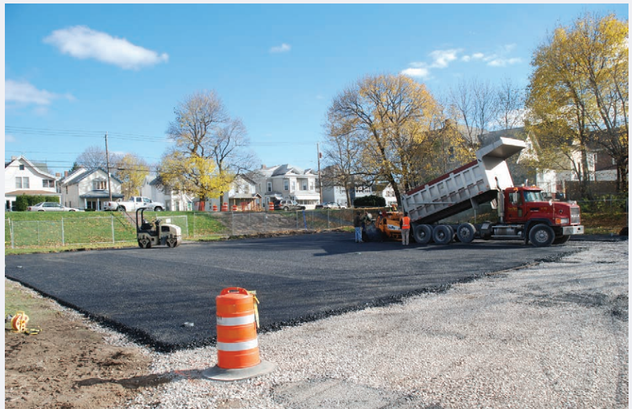
Image 4-CS-3-2. Porous asphalt installation for basketball court.
