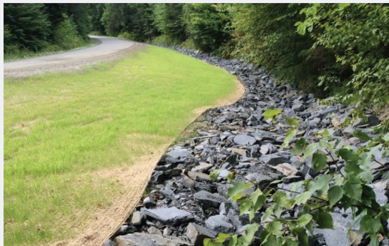
Image 3-CS-2-2. Photo of the project after completion showing the narrower road with vegetated shoulder and stone armored broader, flatter ditch.
