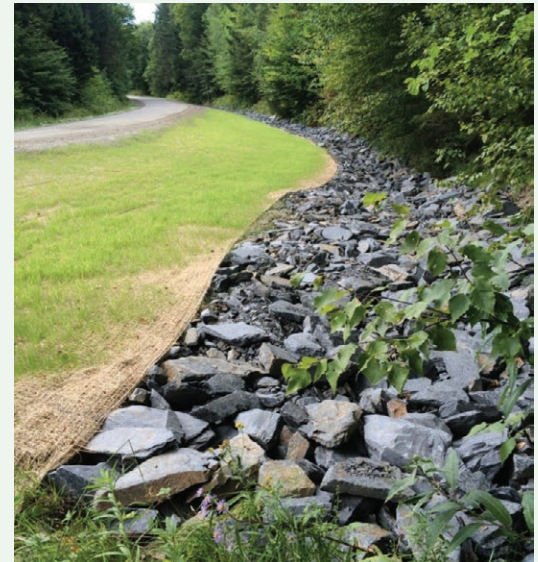
Image PE-8-1. This stone-lined ditch in Vermont is protecting a culvert inlet from sediment clogging.
