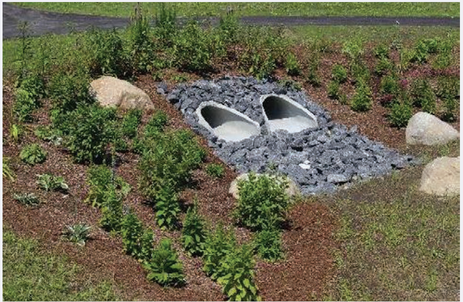
Image 4-CS-2-3. Bioretention inlet with stone armoring to prevent erosion.
