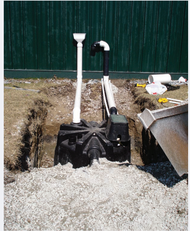
Image 5-CS-3-1. Cistern placement and connection to cisterns.
