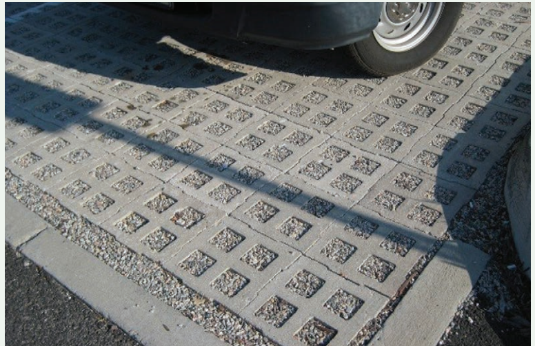
Image PE-13-1. Permeable paver parking installation – light commercial scale.
