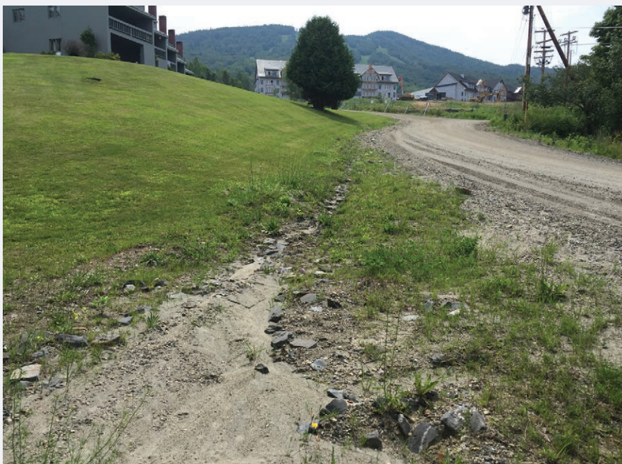
Image 3-CS-1-2. Eroding material from the road surface passes through a formerly stone-lined ditch that is now failing. Below the accumulated sediment is a steep drop to a stream.
