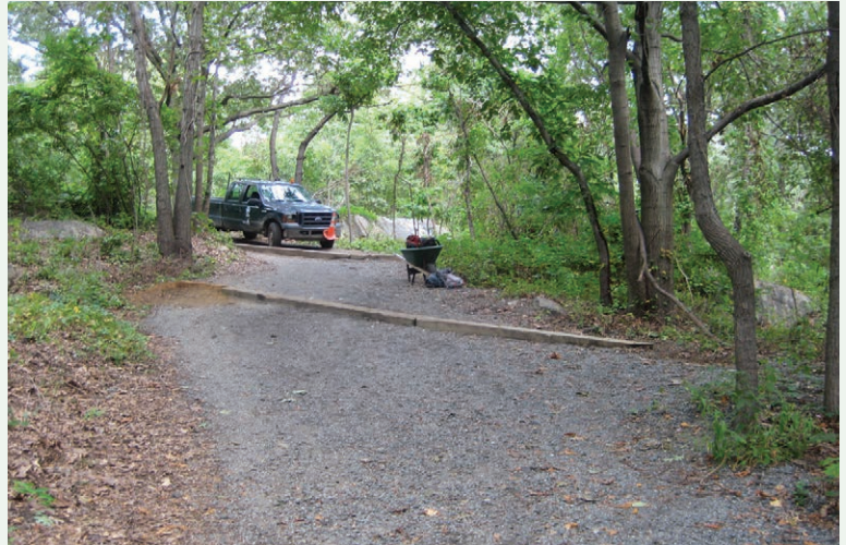
Image PE-10-1. Water bars being installed in Van Cortlandt Park, New York. These water bars will direct stormwater off of this path to the stable vegetation to the side.
