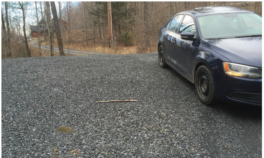
Image 3-2. Roads that have been re-surfaced with either a clean bank run gravel with a high percentage of fine particles, or something like Stay-Mat (crushed ledge product) will tend to hold their shape longer, though construction tends to be more expensive.
