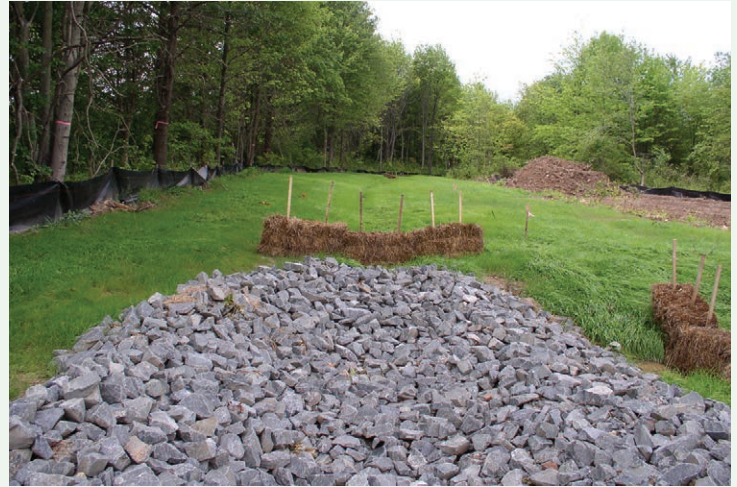
Image PE-6-1. This photo shows an excellent example of outlet protection using larger, well-anchored stones. Hay bales are not part of a permanent solution, but can be useful as temporary velocity controls.
