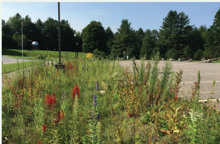
Image PE-2-1. This is an example of a vegetated swale planted with native perennials – though this requires more maintenance than a grass swale, it improves the site. Perennials also say ‘Don’t walk on me!’
