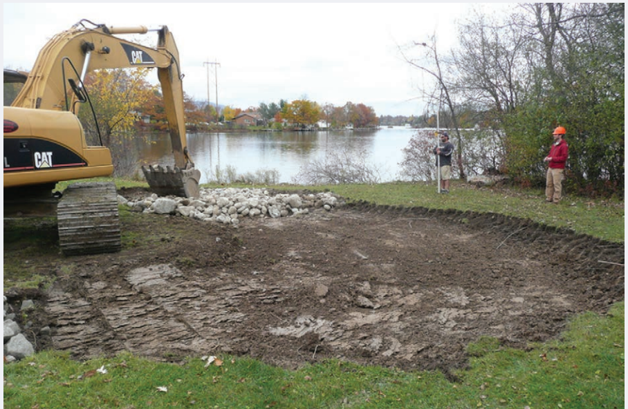
Image 4-CS-4-1. Excavation and installation of rock weirs for the bioretention cell at Mossy Point.
