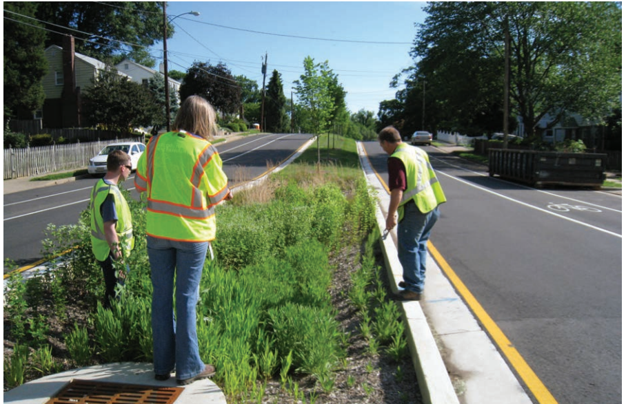
Insert Image 7-1. Municipal staff conduct a maintenance inspection of a bioretention in the road right-of-way.
