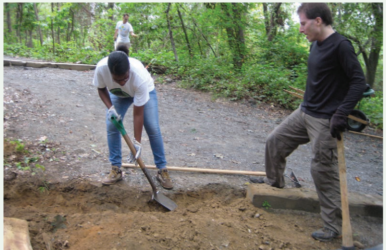
Image PE-10-2. Water bars are easy to install and construction can be completed with just hand tools.
