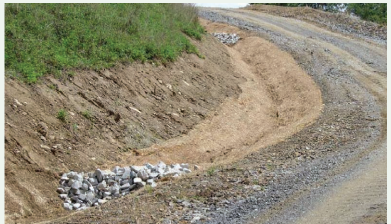
Image PE-9-2. Rock check dams in a roadside ditch in West Virginia with erosion control fabric lining the ditch between them.
