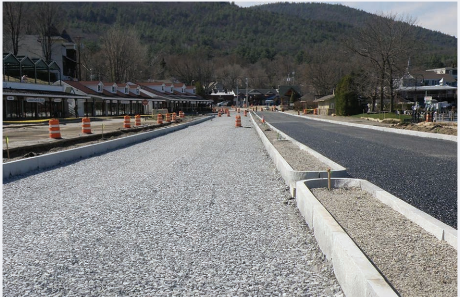
Image 2-CS-1-1. Left lane shows choker stone layer ready for installation of porous asphalt and right lane shows the base course of asphalt ready for the final top course.
