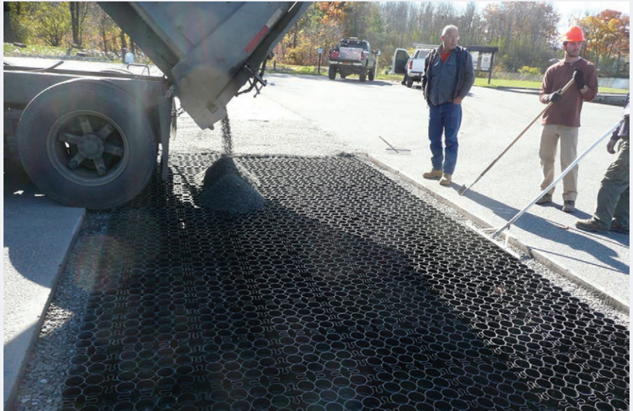
Image 4-CS-4-3. Pea gravel being added to fill the TrueGrid paver mesh in the permeable level spreader.
