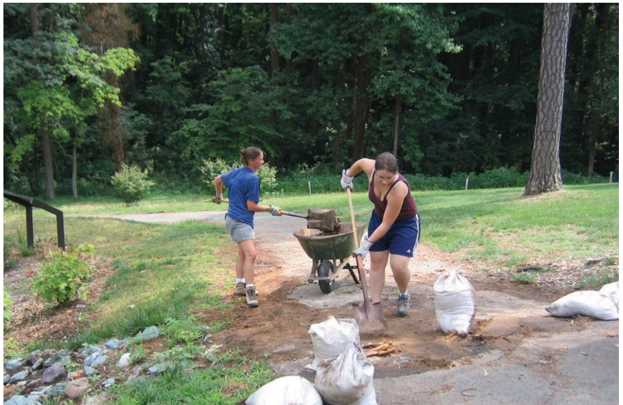
Image 7-2. Sediment removal can often be done by hand.
