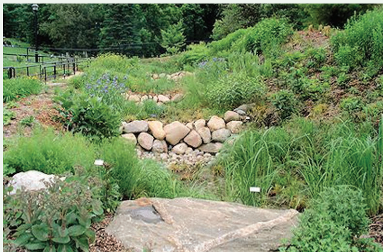
Image PE-2-2. This swale makes use of option check dams to further slow water and filter out pollutants. Use the table to determine spacing.
