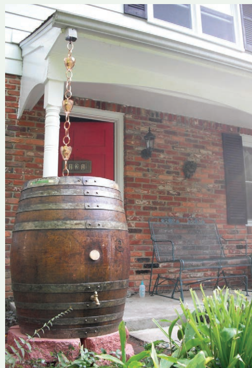
Image PE-15-1. Simple, attractive residential rain barrel using a rain chain to route water from the gutter to the barrel. Note the hose spigot at the bottom of the barrel.
