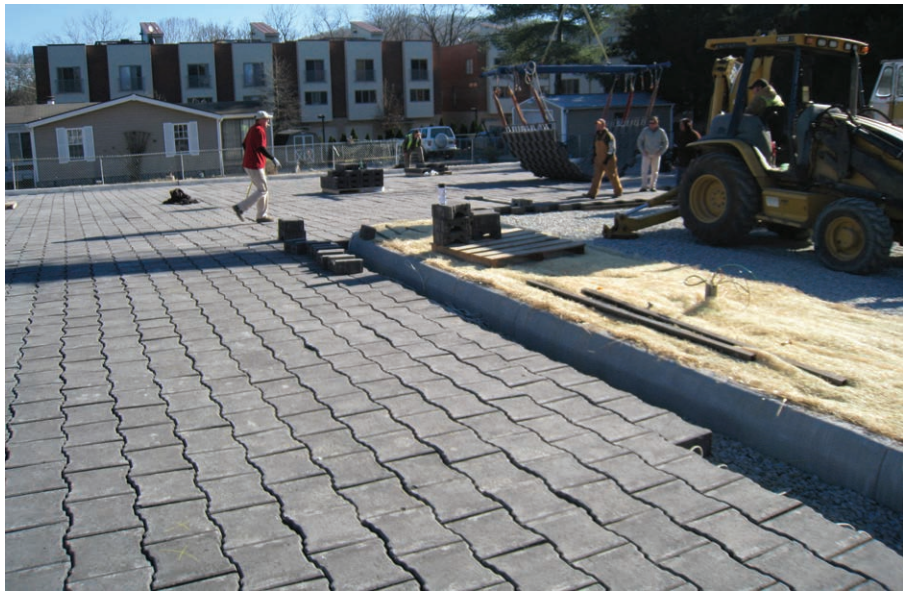
Image 4-1. Permeable paver materials for parking lots and hardscapes come in many styles. They reduce or eliminate runoff from a site by allowing rainfall and snowmelt to infiltrate into the ground below the parking lot.
