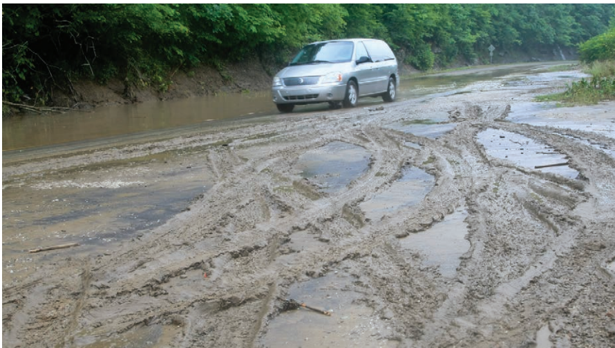
Image 3-1. Some rural roads are built with whatever native soils are at hand, which can lead to the road losing its water-shedding shape and eroding badly.
