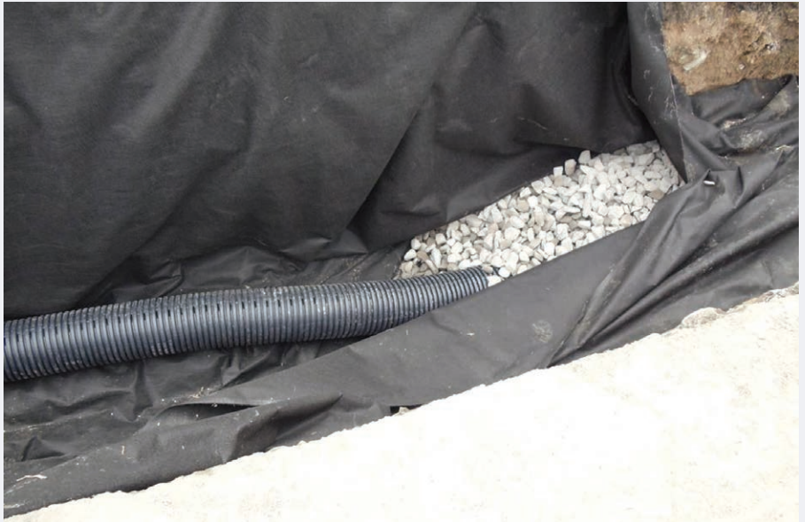
Image 2-CS-4-3. Construction of the underground infiltration trench.
