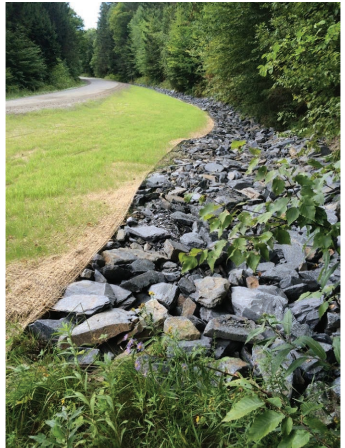
Image 3-3. Stone armoring of roadside swales is often a simple and effective solution to slow runoff and filter out sediment and other pollutants.
