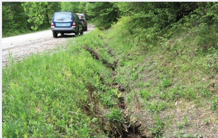
Image 3-CS-2-1. Photo of the ditch along Kew Vasseur road before the project. Note the active downcutting and erosion occurring.
