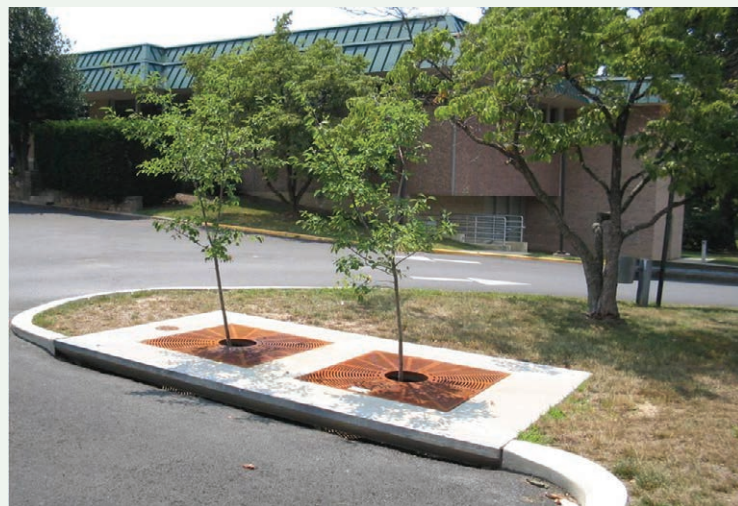
Image PE-3-2. Photo of a dual tree box installation with curb inlet to allow runoff to reach the tree roots
