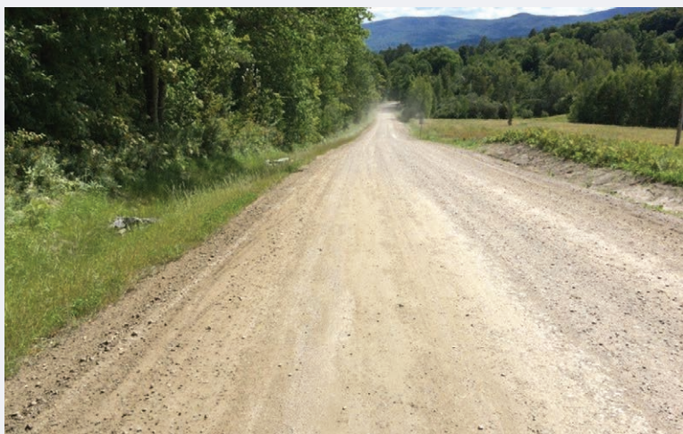
Image 3-CS-2-4. Photo of the project after completion showing the narrower road width with the vegetated roadside swale along the left. One rock check dam is visible in the middle of the photos.
