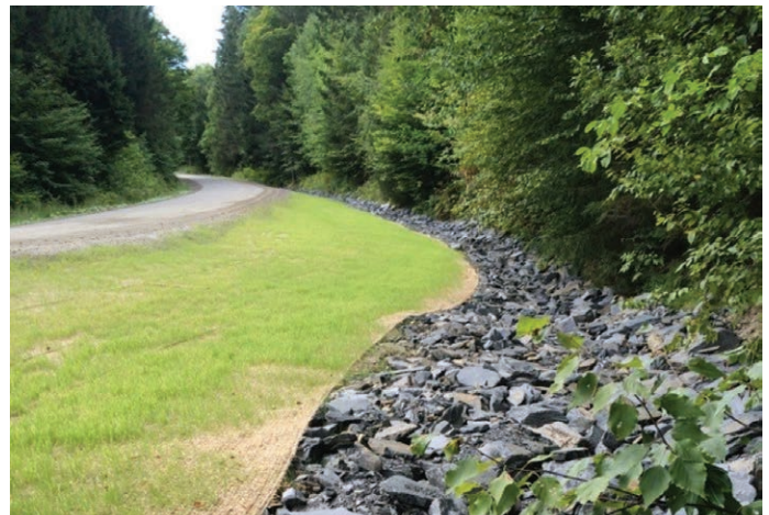
Image 1-5. Stone armoring in rural road ditches can help prevent erosion into water bodies.
