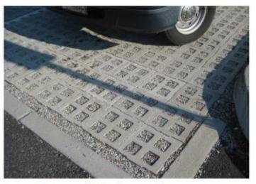
Image 1-3. Permeable hardscapes, like porous pavers, can help manage stormwater runoff.
