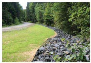
Image 1-5. Stone armoring in rural road ditches can help prevent erosion into water bodies.
