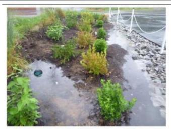
The bottom of the Bioretention cell is not flat, and the water pools at one end, along an edge, or in certain pockets. The whole bottom is not uniformly covered with water. See design plan to verify that Bioretention surface is intended to be flat. Check during or immediately after a rainstorm.
