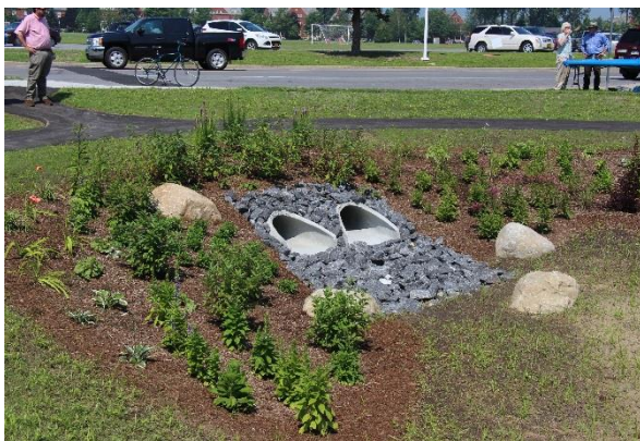
Figure 5-17. Photo of bioretention basin inlet
