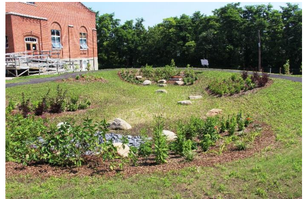
Figure 5-16. Photo of bioretention basin
