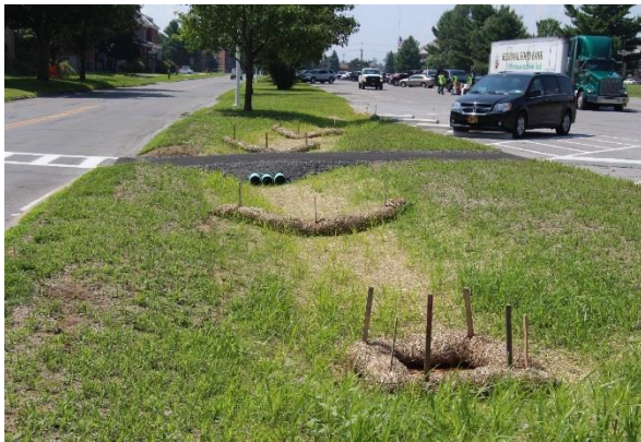
Figure 5-15. Photo of bioswale
