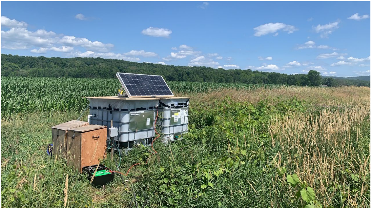
Figure 9. The original experimental design setup with the filter units, ISCO samplers, solar panel, batteries, sump, and the Sunpump.
