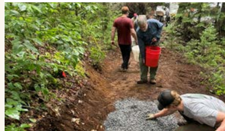
Reducing cross slopes, preventing erosion, and improving user safety along 100 feet of Northern Forest Canoe trail.
