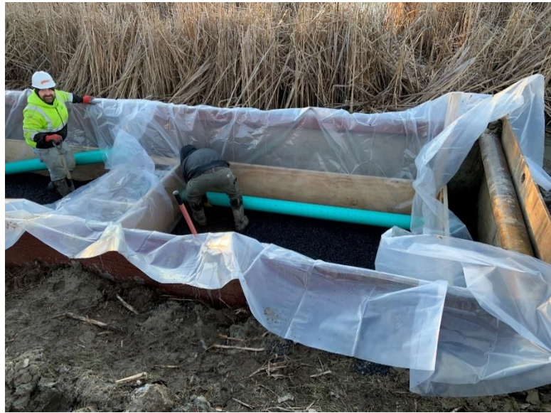
Figure 1. Installing perforated distribution pipe in Filter F_{AA}
