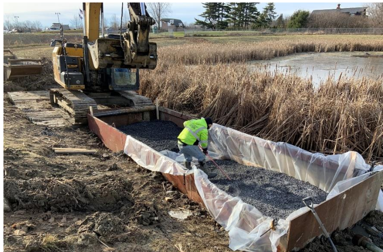
Figure 2. Raking top of media bed
