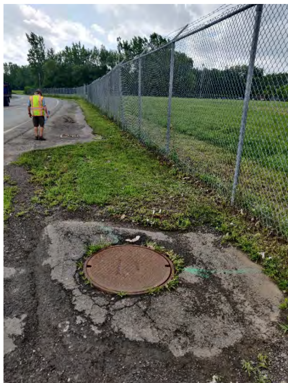
Figure 10. Sanitary manhole SAM01
