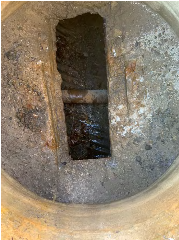
Figure 6. Sanitary sewer lateral crossing Elizabeth Street stormdrain
