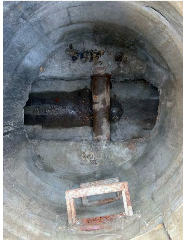
Figure 7. Sanitary sewer lateral crossing Johnson Street stormdrain
