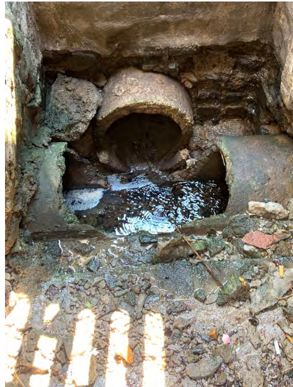
Figure 17. Foam in PB31 catchbasin CB07
