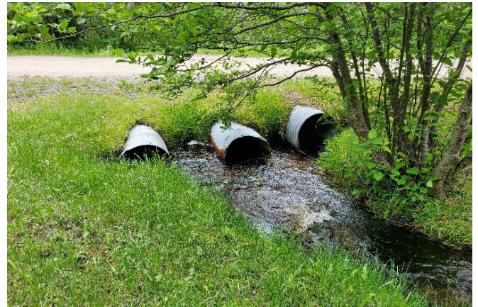
Inlet to Goldsmith Rd crossing –TU, 6/13/2023
