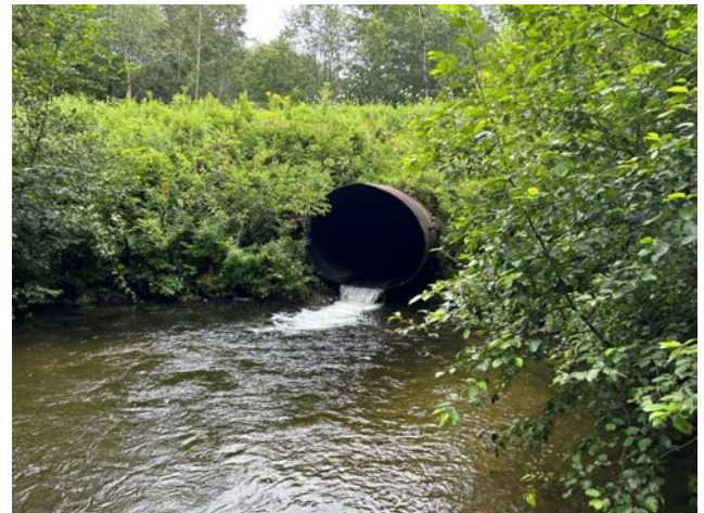
Joess Brook Culvert Outlet, Downstream
