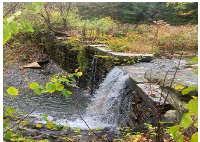
Pelletier Dam is targeted for removal
