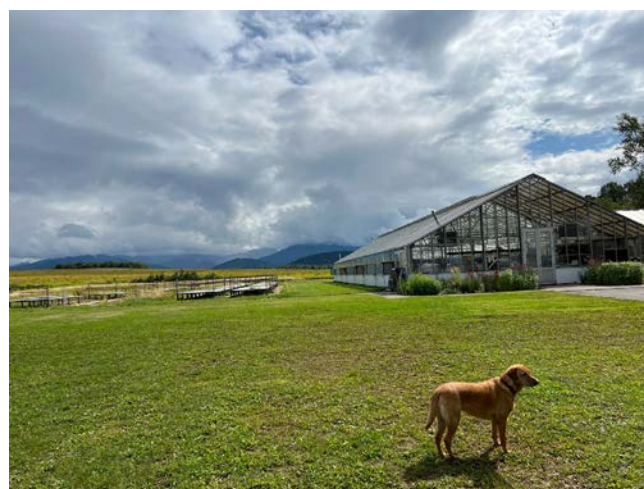
The current greenhouse stands to the right and will see significant upgrades. Immediately left are the old plant benches with the existing foundations to house the new high tunnel.
