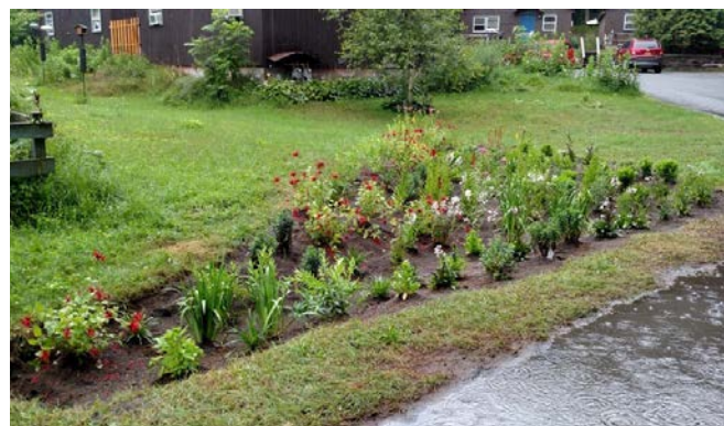
Past project - bioretention area / rain garden.
