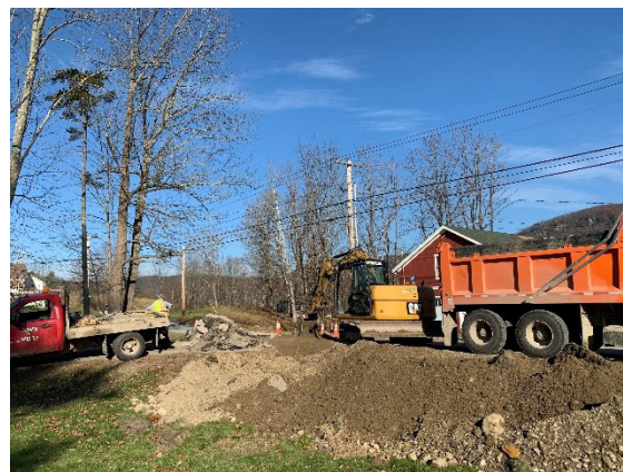
Stormwater project implementation in Wells, VT
