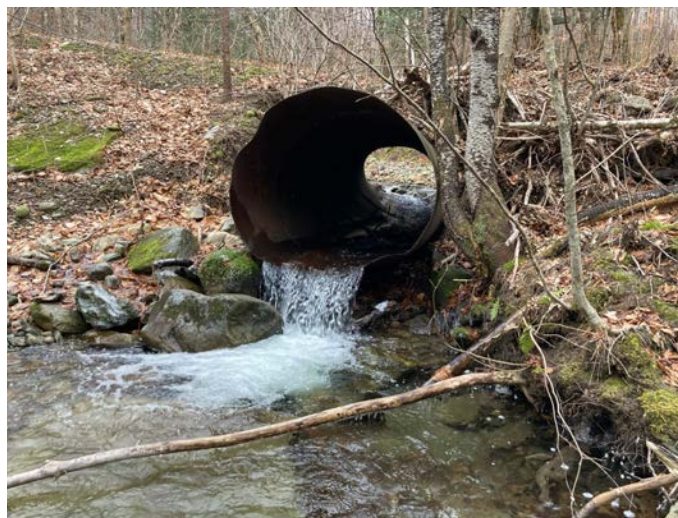
Undersized, perched culvert on private maple sugaring land in the Missisquoi River basin (Bakersfield, VT).
