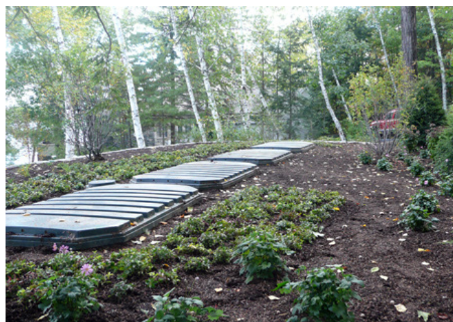
Completed septic installation.
