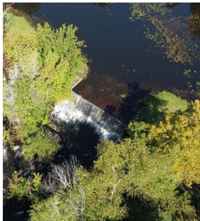
Aerial view of the Penfield Pond Dam.
