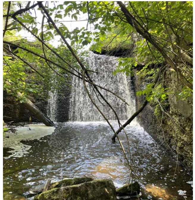
Trout Brook Reservoir Dam with water flowing over the spillway in September 2022.
