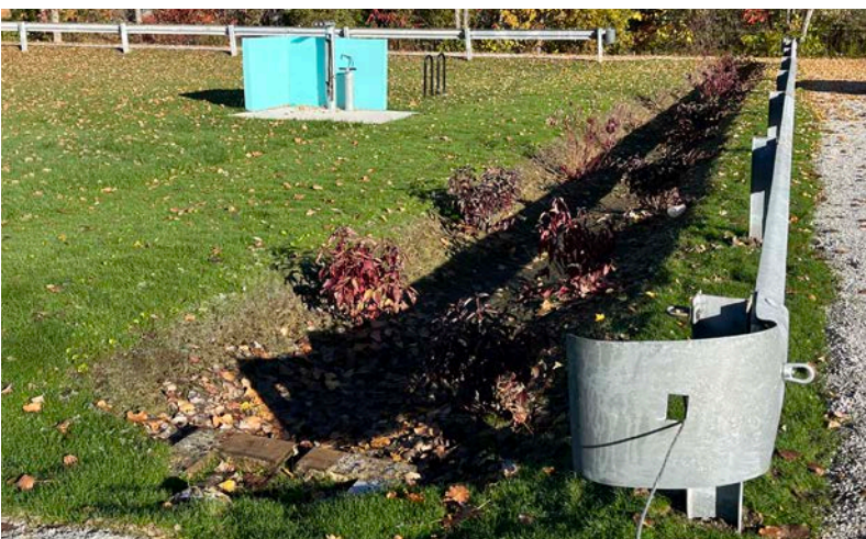
Completed stormwater bioretention area off of Swanton Beach parking lot.
