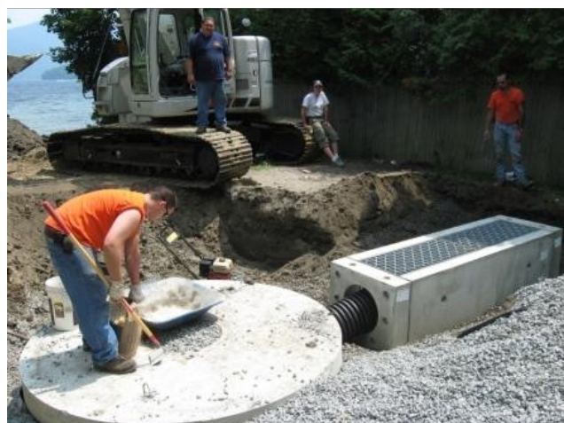
Past Project: Dry well and trench drain installation (not at POV).
